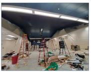
The damaged wood and concrete flooring in the gym has been removed. Once the downstairs has been
